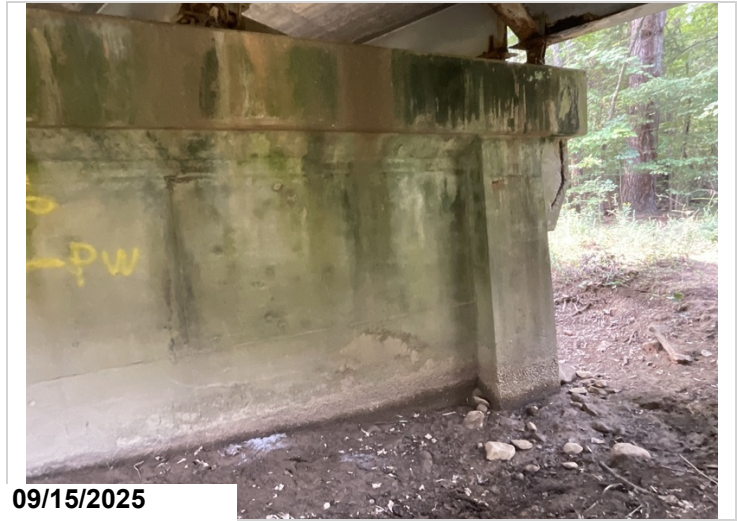
Bent 4 backside right has 1lf exposed rebar cs3 and abrasion to lower exposed portion
