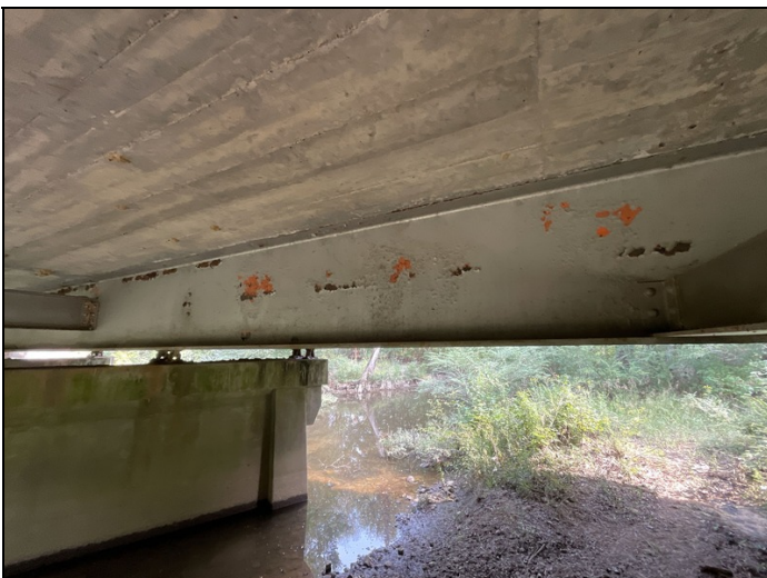
All beams have scattered areas of corrosion
