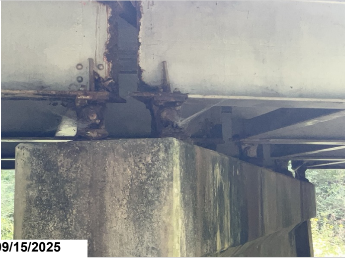
Bent 4 bearings
