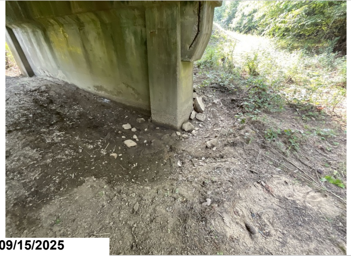
Bent 4 right side has a 3' deep by 10' around horseshoe scour
