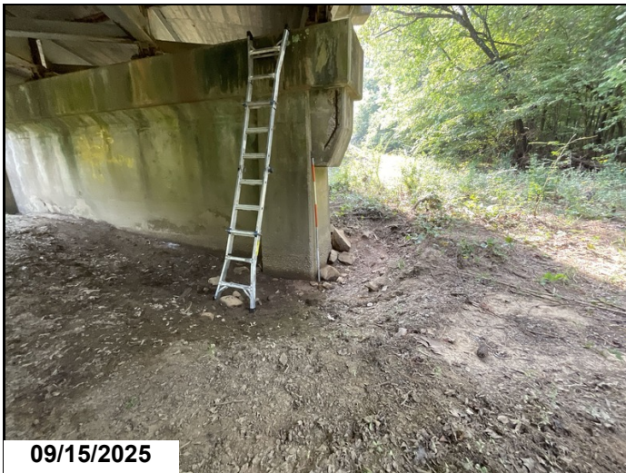
Bent 4, right side: local scour action removing material away from pier. Similar condition to bent 3.
