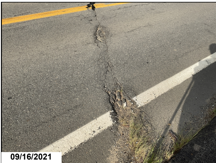
Bent 4: asphalt overlay with a pot hole at the joint in the westbound lane.
