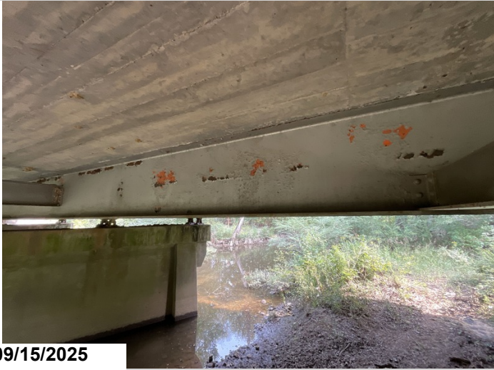
All beams have scattered areas of corrosion
