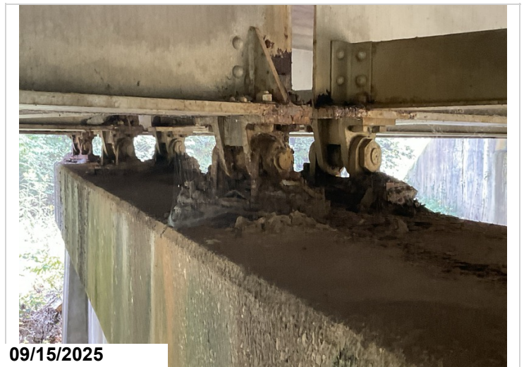
Girder ends and bearings are in need of major cleaning and repairs
