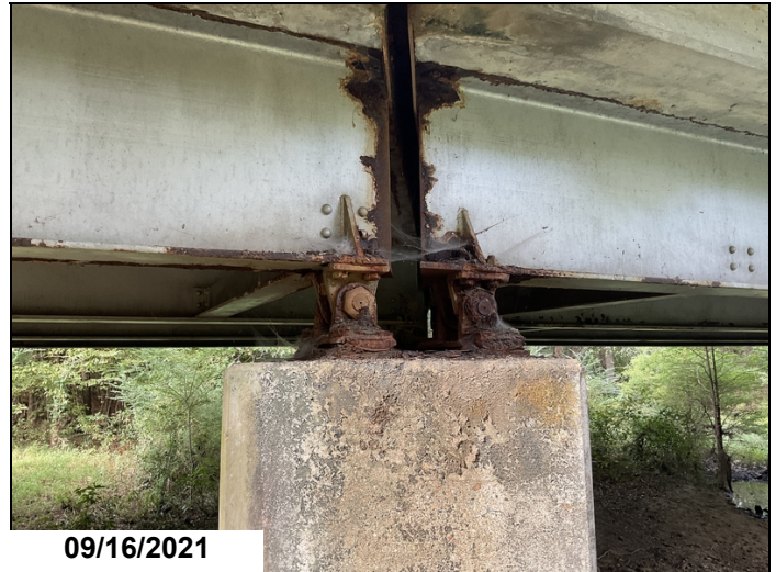
Bent 4, spans 3&4, girder 1: both bearings and beam ends with laminating rust with section loss.
