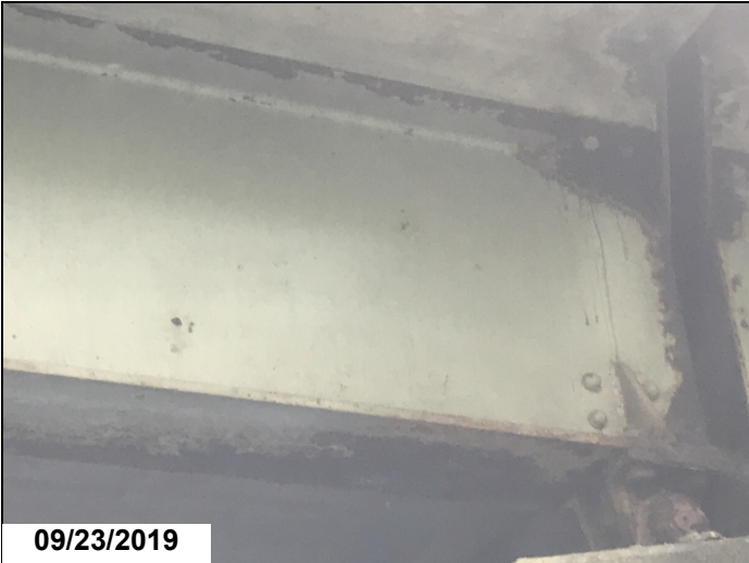
Span 2 beam 4 at bent 3 active corrosion on the beam end with moderate pitting.
