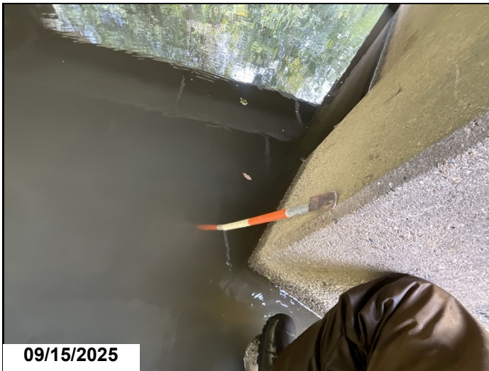
Bent 2 upstream end, 4' deep scour hole exposing footing. Footing is not undermined at this time.
