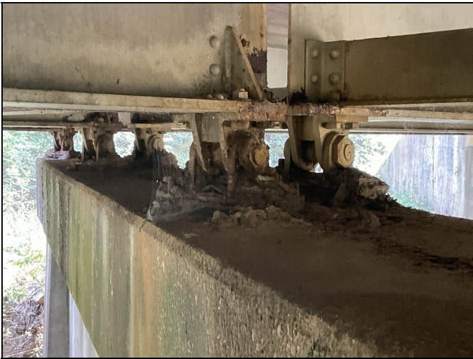
Girder ends and bearings are in need of major cleaning and repairs
