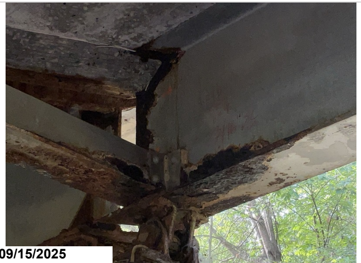
Bent4 girder 4 has up to 1/4" section loss to lower flange
