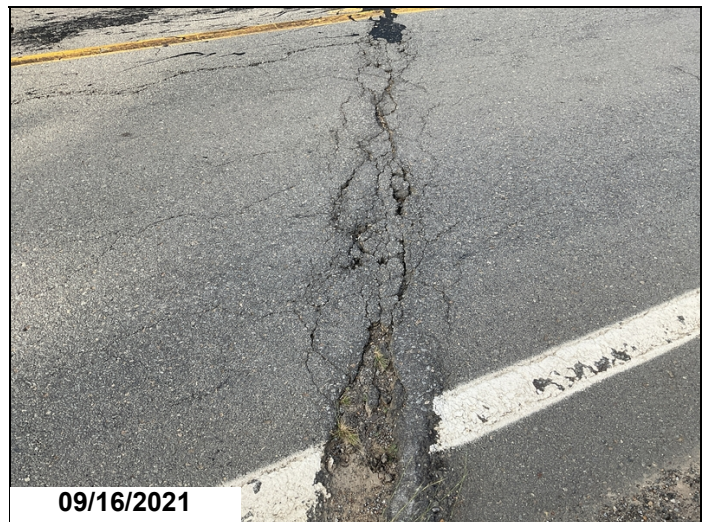
Bent 2: asphalt overlay with a pot hole at the joint in the westbound lane.
