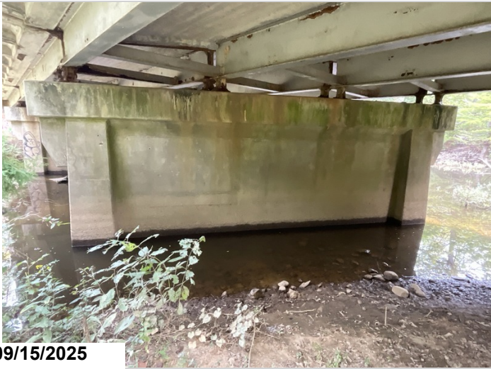
Columns have abrasion to lower exposed portions
