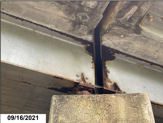
Bent 3: active corrosion on the beam end with moderate pitting.
