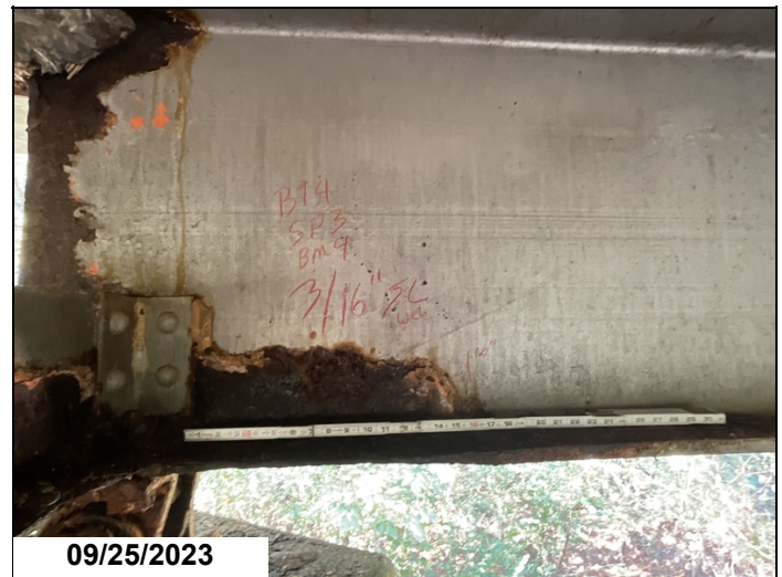
09/25/2023 span 3, at bent 4 beam 4, 1/4" remain on left side of bottom flange. Up to 3/16" section loss in lower web. Worst case this bridge.
