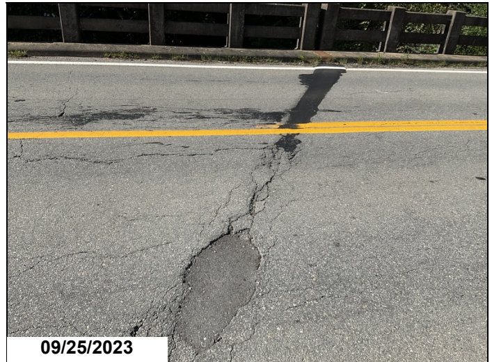
Bent 2 potholes have been patched
