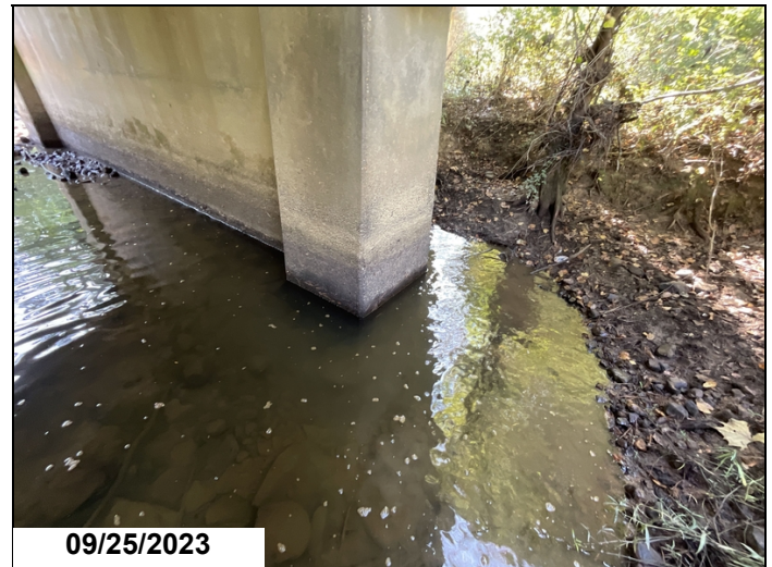
Bent 3 upstream end, local scour has exposed top of footing
