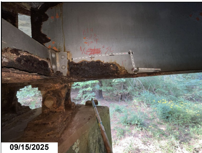
09/15/2025 Bent 4 span 3 girder 4 1/4" section loss to lower web and bottom flange
