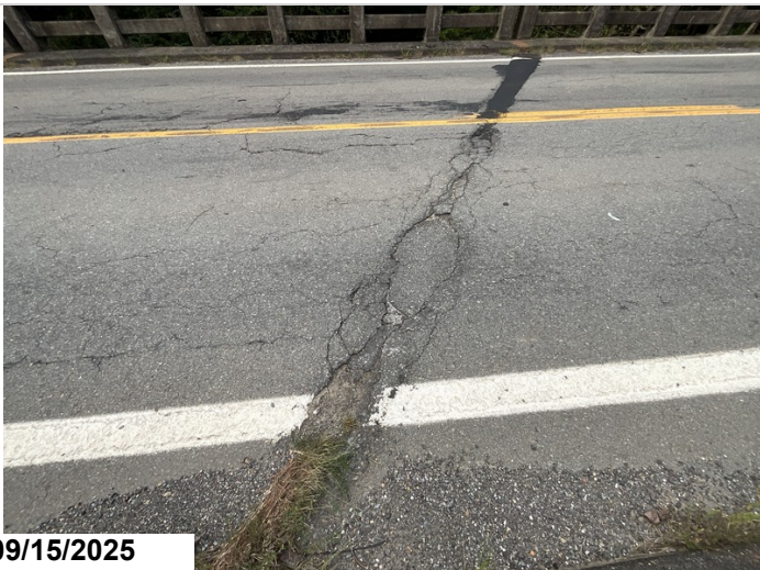
Potholes at bent 2 in asphalt overlay
